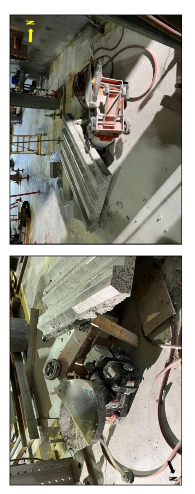
Figure 6.8.12: Husqvarna floor saw trapped under a portion of the collapsed concrete slab.
