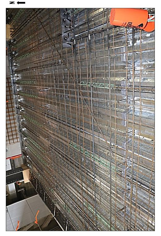
Figure 6.9.21: (a) Construction image showing the rebar reinforcement of the northwest corner of the CF Project test frame.
