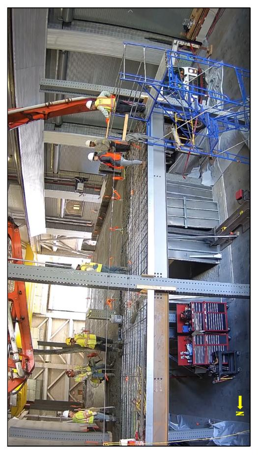
Figure 6.4.20: Construction image showing the concrete decking installation.
