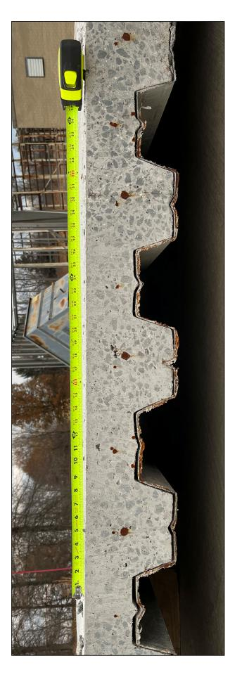
Figure 6.9.5: Typical cross-section of the composite floor. Shown in this image is the south cut face of Slab 1.
