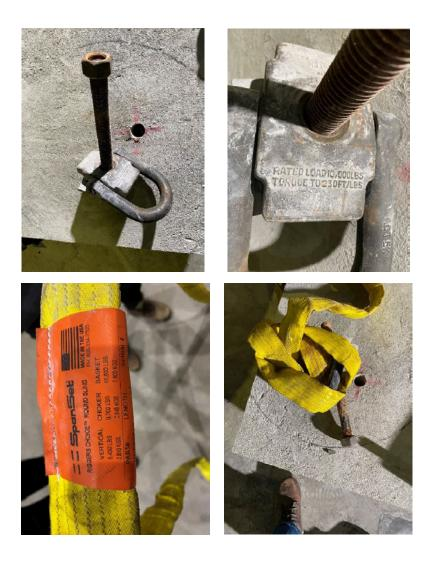
Figure 4-2 – Drilled hole for anchoring sling, load capacity marking on anchor, sling attachment as choker, marking on sling showing a capacity of 3,040 kg (6,700 lbf).
